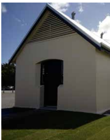
The refurbished Dairy.
