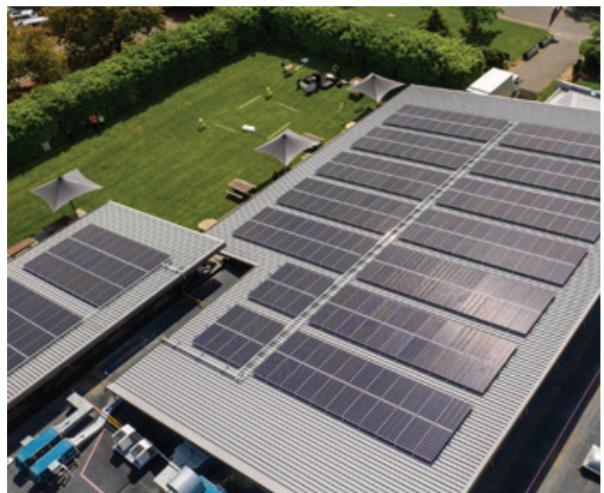
The first of the planned solar arrays on campus, Te Kete Ika solar array was completed in November 2019.
